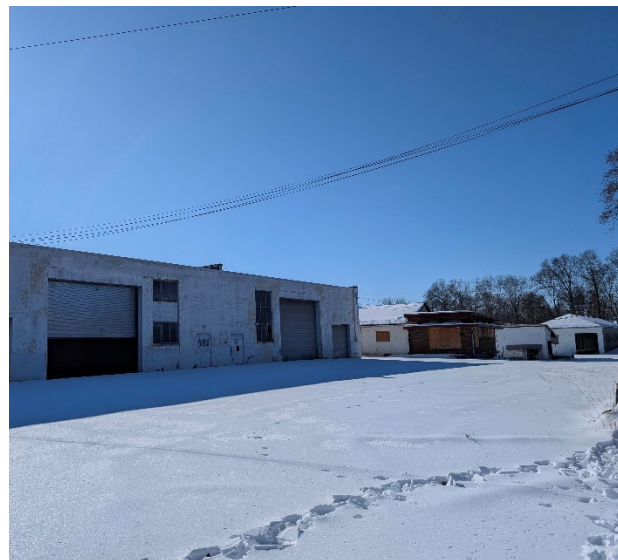
View of Building A (left) and Building B, C and E in the background (right). The above images show boarded up windows and broken garage doors.
