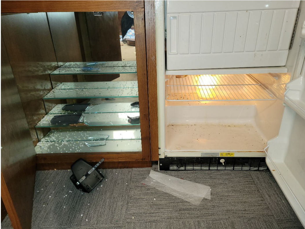
View of the still functional mini-fridge in the office with the door open showing rodent droppings.
