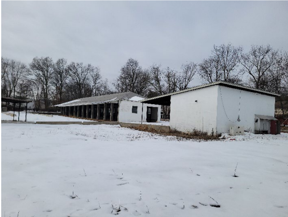
View of the exterior of Building C (foreground) and Building E (background)
