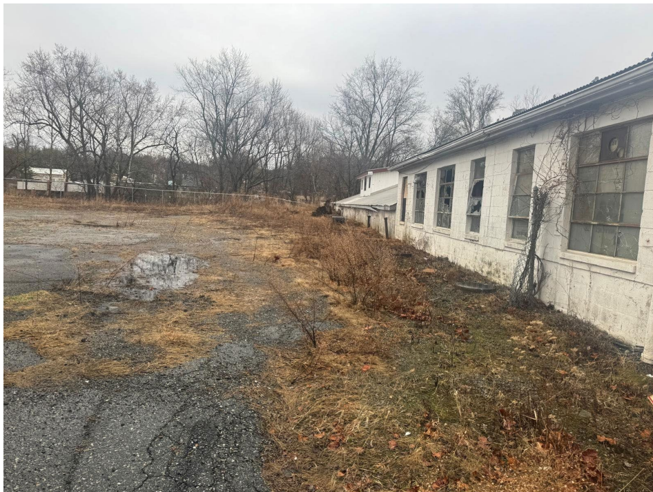
View of the northerly side of Building B and the northeasterly corner of the property. This area is characterized by poor drainage, deteriorated asphalt, and overgrowth.
