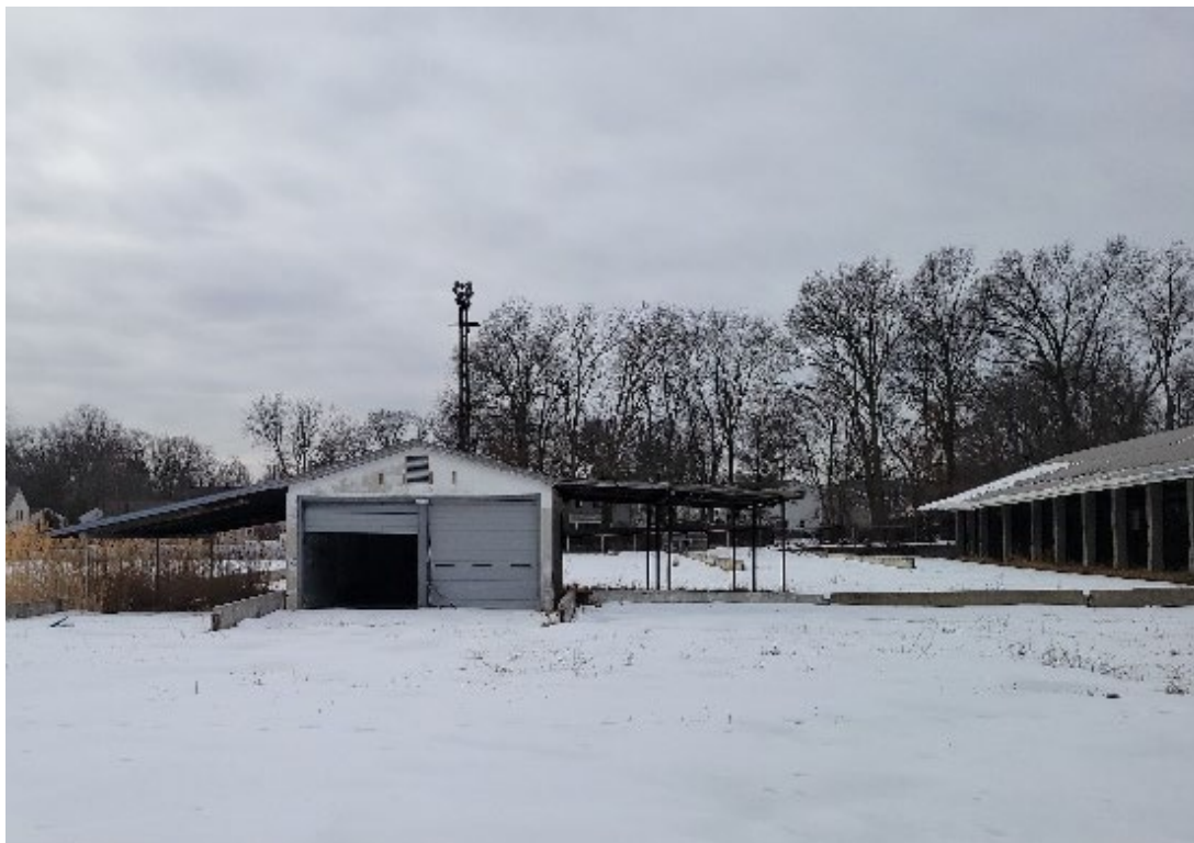
View of Building D and the yard to the rear of the same. Building E is also pictured (right), showing the cinder block pillars without the walls.
