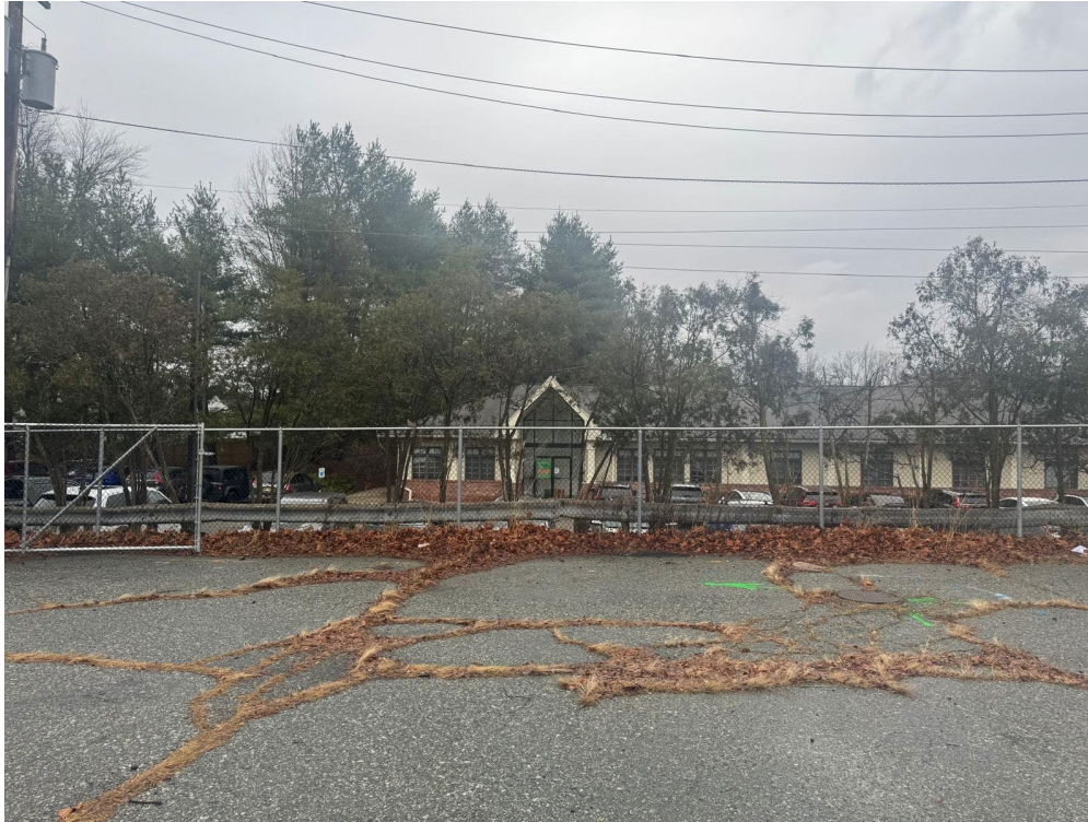
Additional view of the cracked pavement and the chainlink fence along the northerly property line. Also pictured is the commercial building on the adjacent property (271 Grove Avenue).
