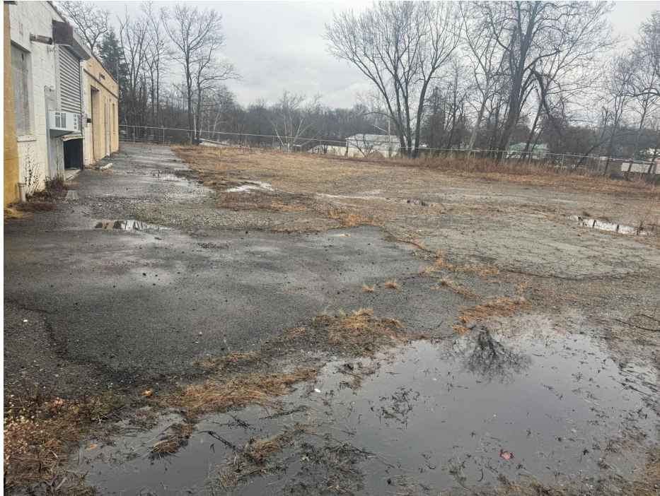
Another view of the rear of Building A and the northeasterly corner of the property, showing pool of water (just after a rain event) and significantly deteriorated asphalt.
