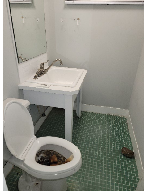
View of another bathroom located in Building B.
