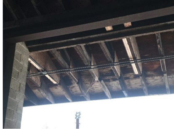
View of the roof overhang that is located above the columns.
