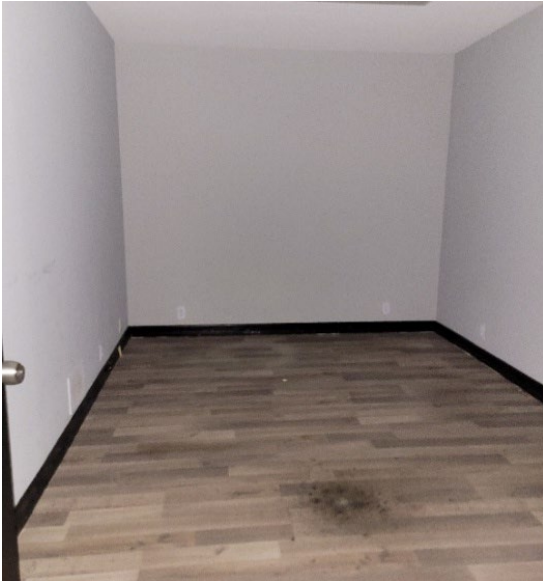
View of a room in the office space, bearing evidence of a small fire suggesting acts of vandalism.
