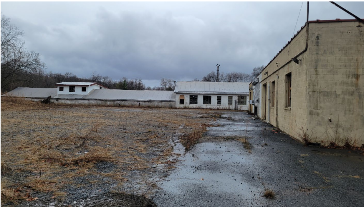
A view from the rear of Building A with Building B in the background. The ground in this area is muddy and covered in broken asphalt and gravel.
