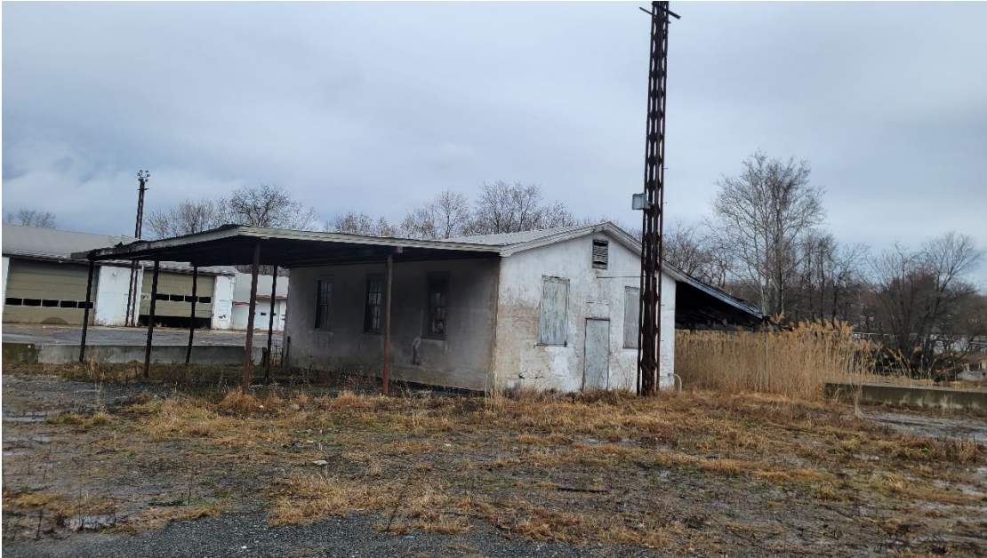
Another view of the southerly side of Building D with boarded windows.
