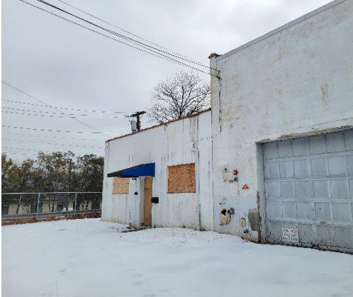
View of the boarded-up entrance to Bldg. A.
