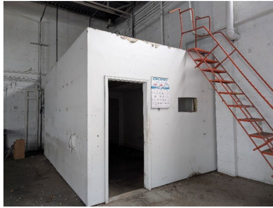
View of an office space in the garage.
