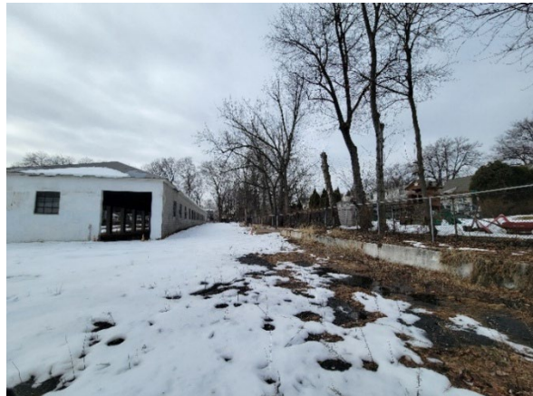
View showing how close Building E is to single-family homes.
