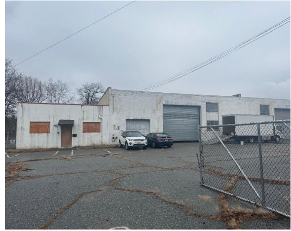
View of Building A from the entrance gate. The pavement is cracked with overgrowth.
