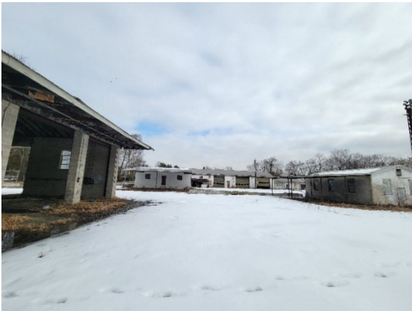
View looking at Building E to the left with buildings C and B in the background and D to the right.
