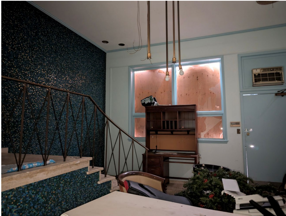
View of front lobby of Building B with pile of garbage and furniture.
