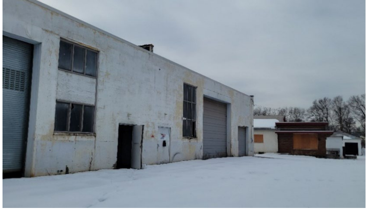
Another view of Building A's garages with clerestory windows.
