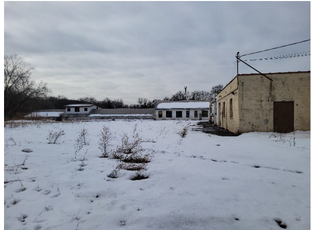
View to the rear of Building A (tan) and side of Building B (white) taken from near the northerly property line.
