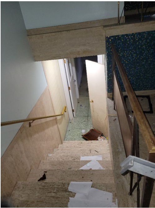
Staircase to the upstairs offices. Broken glass and debris can be found on the floor.
