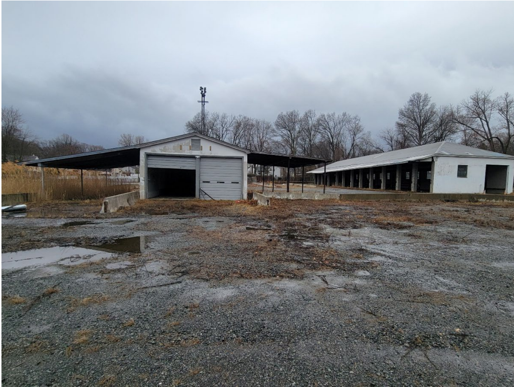
View of Building D with a pool of water in front of the building indicating the deteriorated pavement and inability to drain stormwater.
