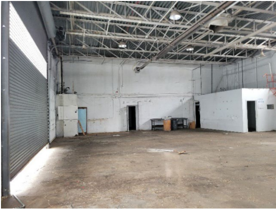
View of the garage along the front of the building
