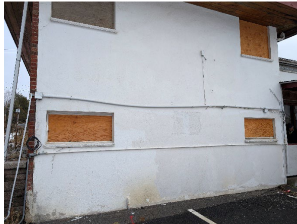
Additional view of the side of the building that shows more boarded up windows.
