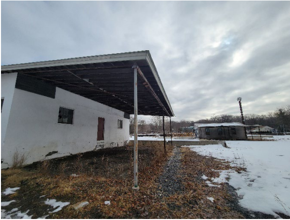
View of the side of Building C
