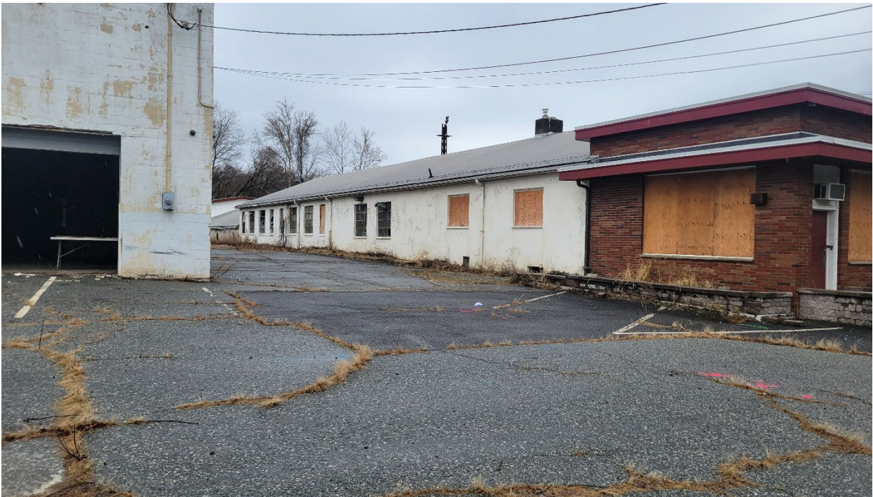
A view from the front of Building A (left) with the garage bay open and the front of Building B (right) with the boarded-up windows.
