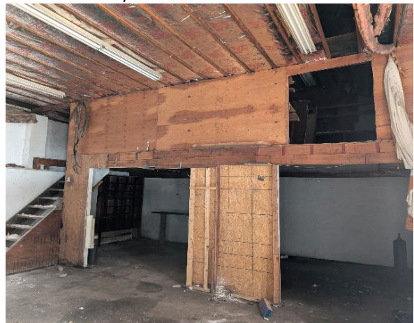
Front-facing view of the loft and the area below it.
