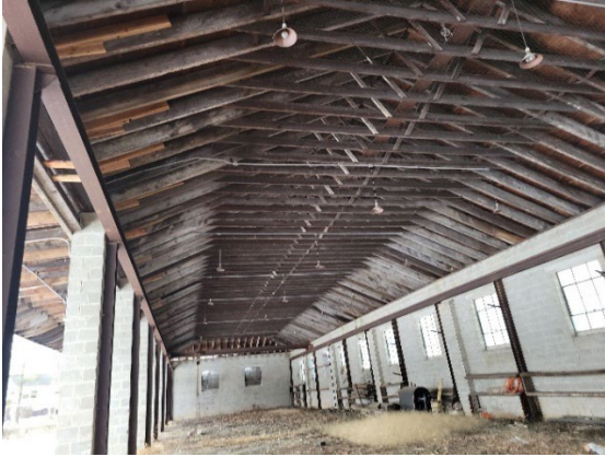
Interior view of the partially enclosed A-Frame building
