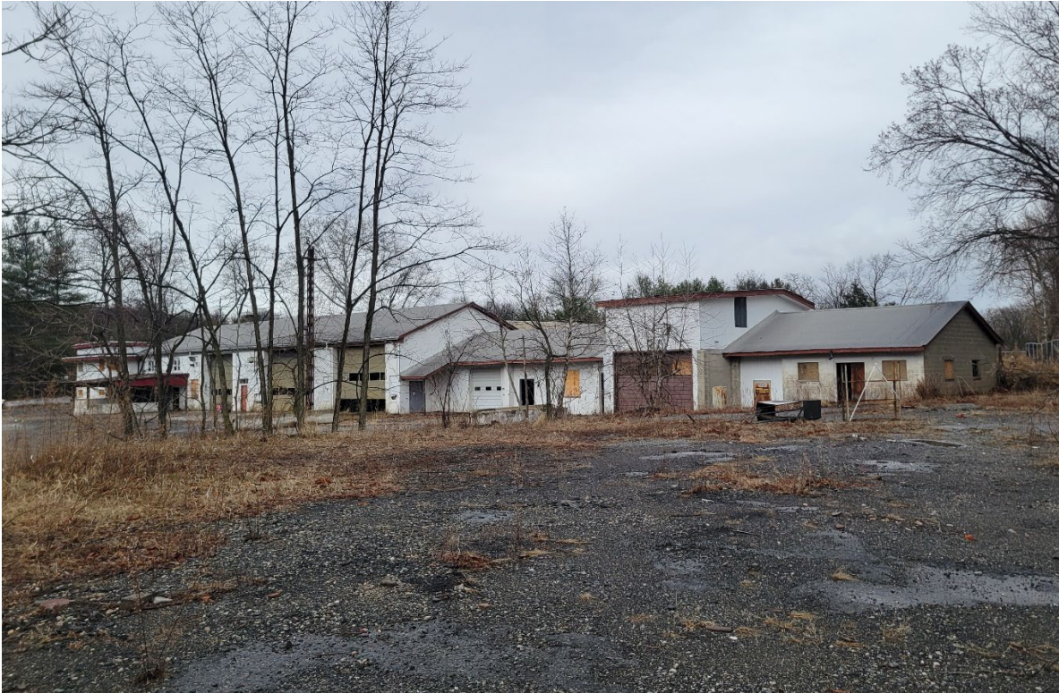
A view of the rear portion of Building B from the easterly property line. The rear of the building contains three large garages and several attached storage rooms.
