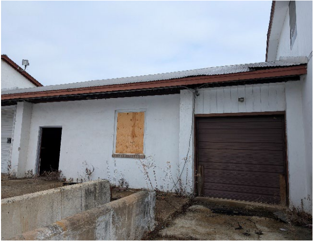
View of more rear entrances to the building with a boarded-up window.
