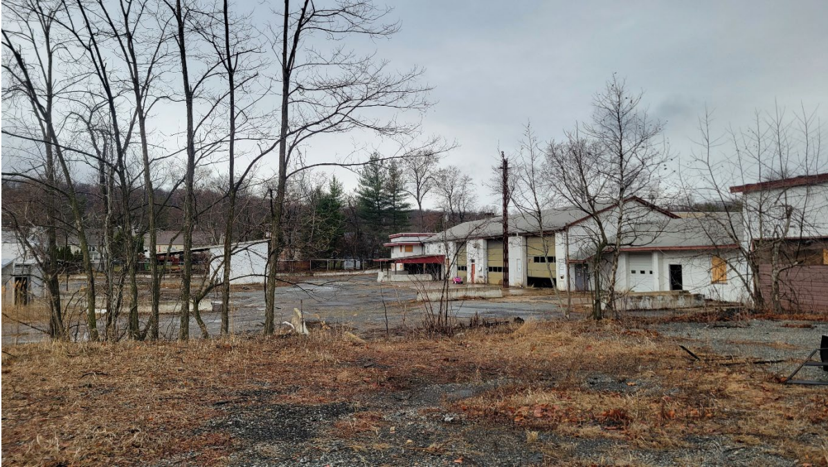
Another view from the easterly property line. Building C is in the center and Building B is to the right
