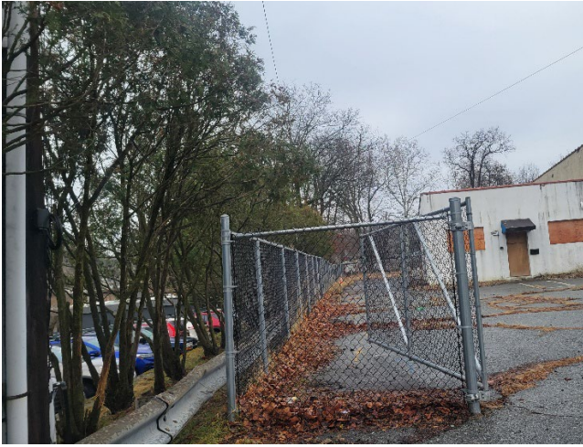
View of northerly side of Building A and the chain link fence that encloses the property.
