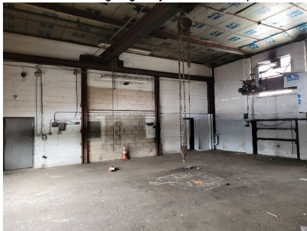
View of a third garage bay with debris on the floor.
