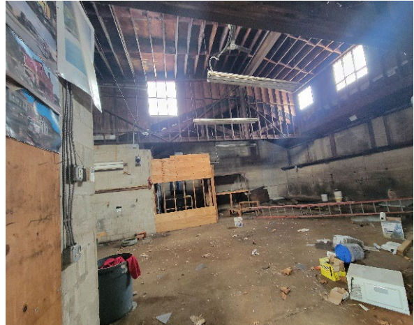
View of the fourth garage bay with debris and abandoned equipment by the previous tenants.
