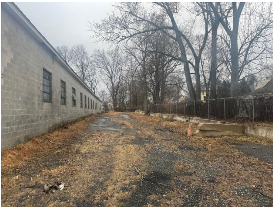
Close up of Building E with respect to the residential homes.
