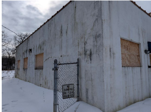
View of boarded up windows along the front and side of the building.
