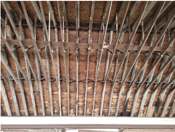
View of Building E's ceiling that includes a wiring mesh.
