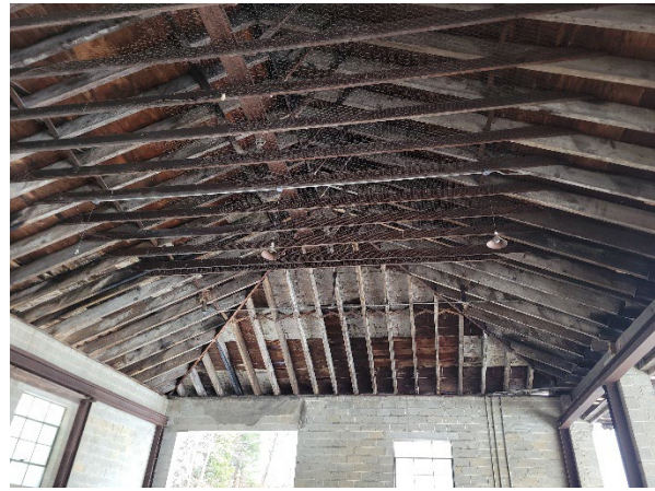
Additional view of Building E's ceiling.
