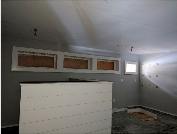
Office space located in Building B.
