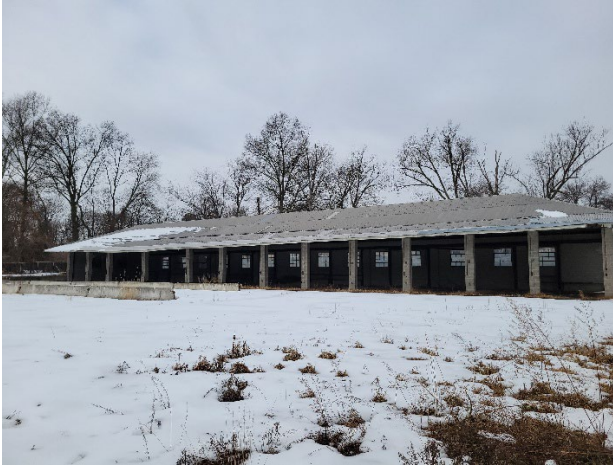
Exterior view of Building E with the twelve (12) openings.
